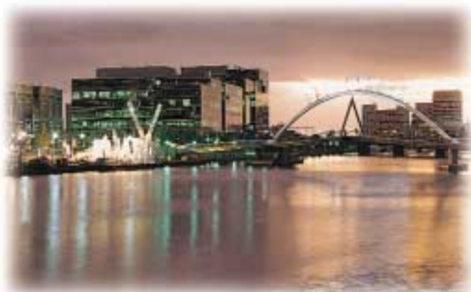
At Healesville (Victoria) the town's wastewater is disinfected with UV prior to entering the Yarra River which flows through Melbourne.
